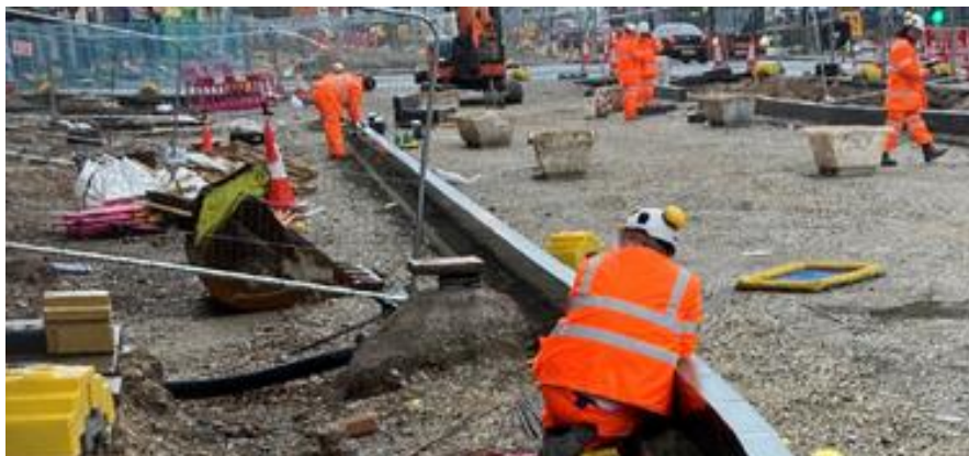
Figure 17: West Midlands team performing essential mains replacement works
