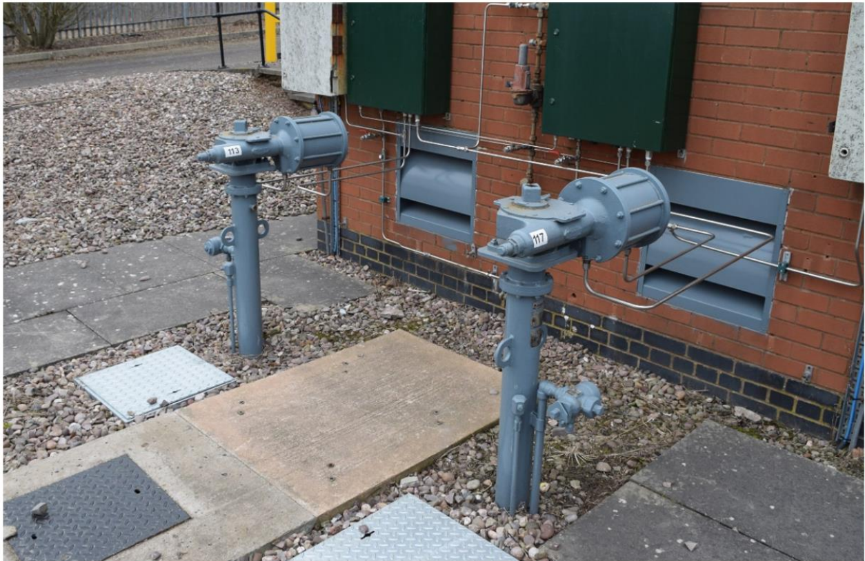
Figure 5: Audco Actuator associated with Slamshut
